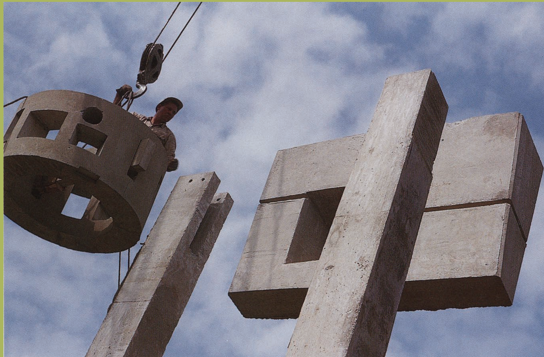
Each sculpture was cautiously hoisted by a ten-ton crane into its slotted footing.
